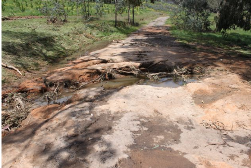
Figure 5: Stream crossing damage – Coppabella Station (MV), October 2011.
