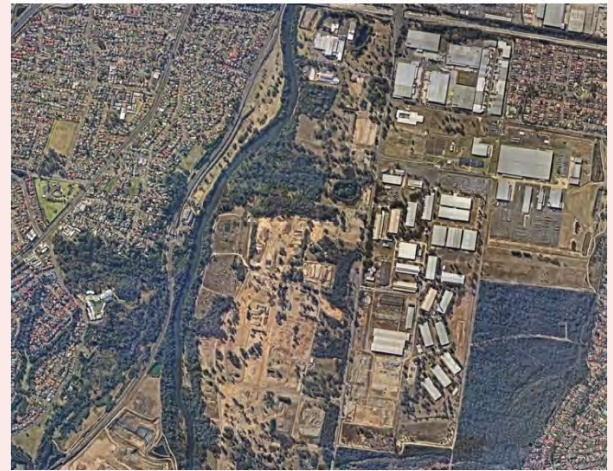
Moorebank Intermodal construction progress at August 2017
