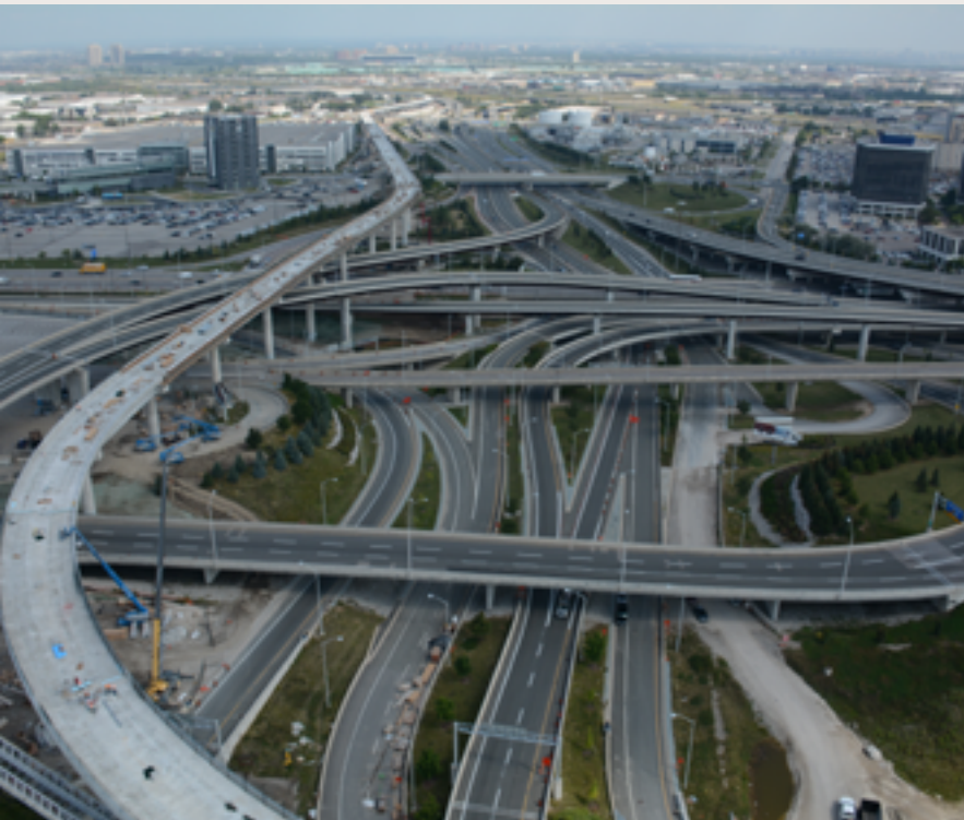
Construction on the Union Pearson Express airport rail link rises above highways.
