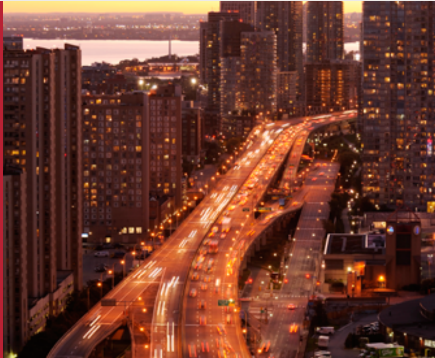
The Gardiner Expressway and downtown Toronto.
