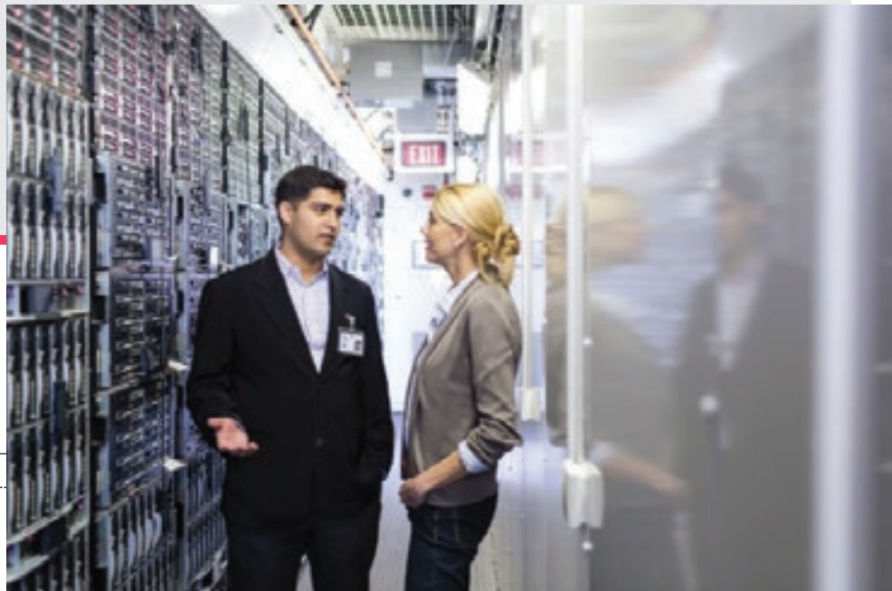
HP Data Centre
